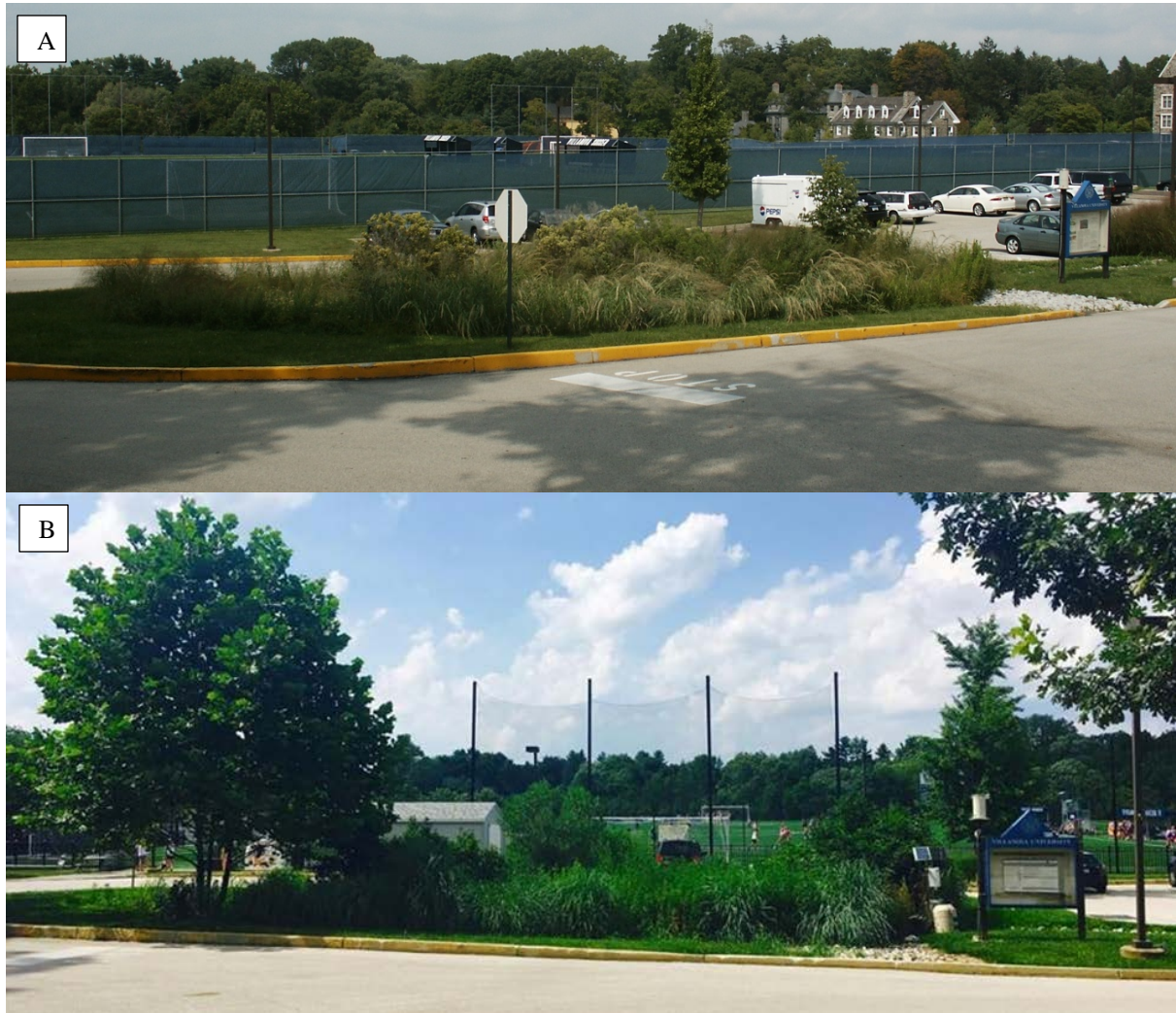
Figure 1. A.) Photograph of VU Bioinfiltration Rain Garden BMP (2007). B) Photograph of VU Bioinfiltration Rain Garden BMP (July 2017). The site has matured over time with volunteer plant species inhabiting the site along with planned plantings.
